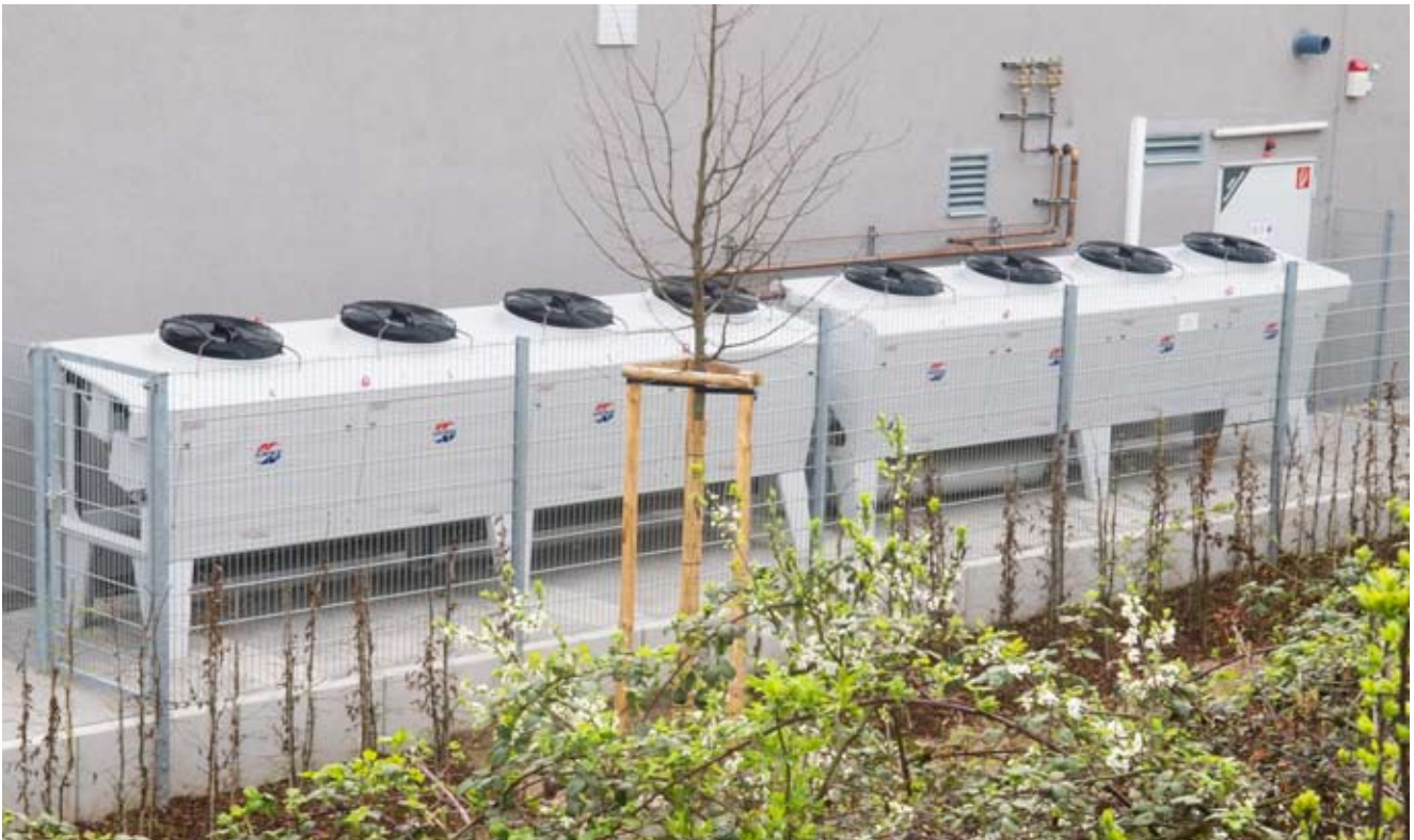
The GVX condensers have EC fans.
