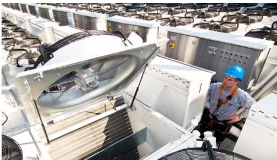
The hinged fans make cleaning easier
